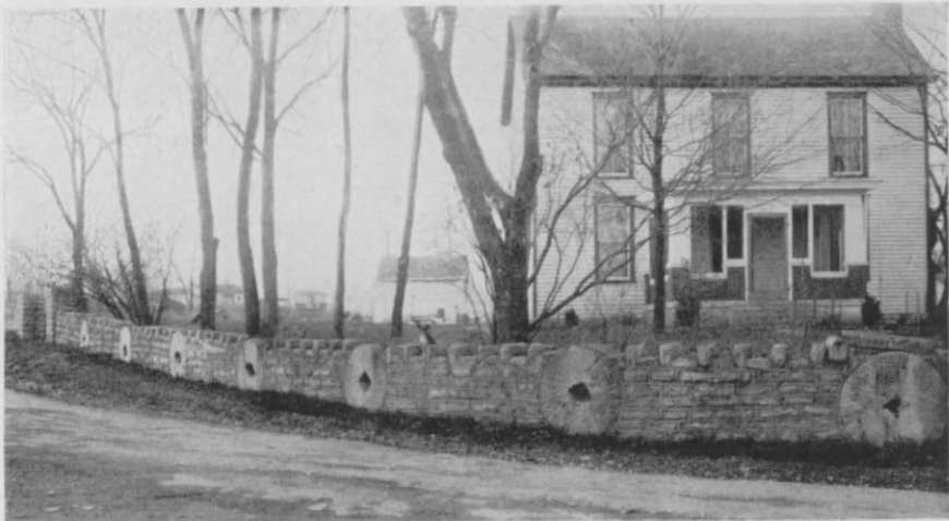
8. Old millstones from the Weisenberger Mill, in Scott County near Midway, were used in the construction of this stone fence. It is just across the road from the old mill, at the home of the present miller who is a lineal descendant of the first miller at this site
