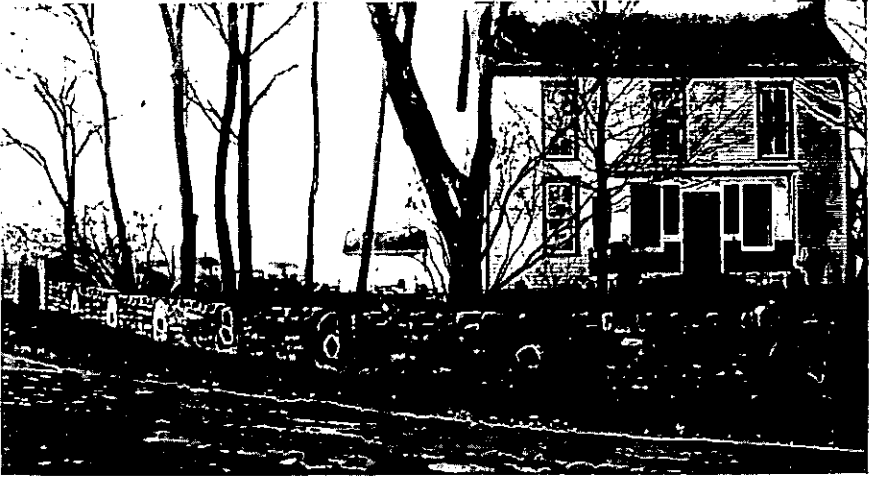
8. Old millstones from the Weisenberger Mill, in Scott County near Midway, were used in the construction of this stone fence. It is just across the road from the old mill, at the home of the present miller who is a lineal descendant of the first miller at this site
