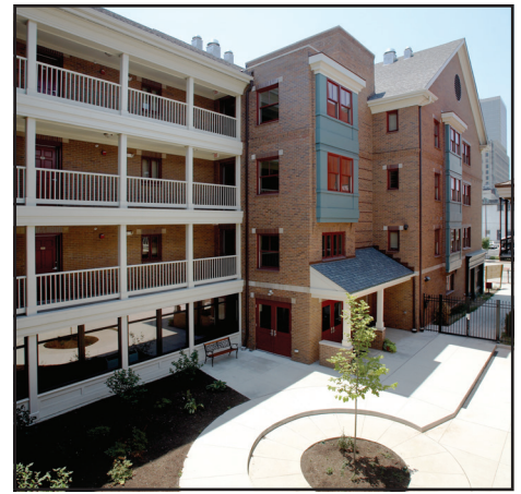
Charles Raith, 1952-. Architectural Papers, circa 1970s–2010 [Mss. AR R161a] The shared courtyard of the Howard-Hardy House and the Cathedral Commons Apartments.
