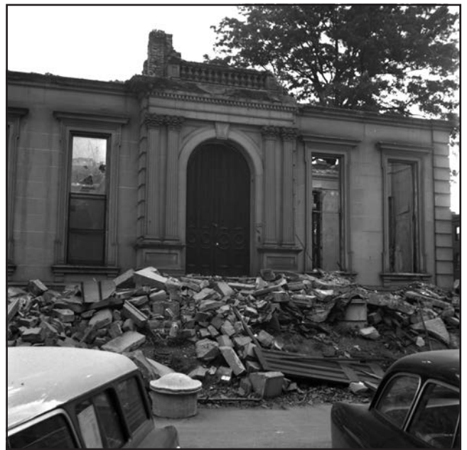
View of building at 924 South 4th Street being torn down.
