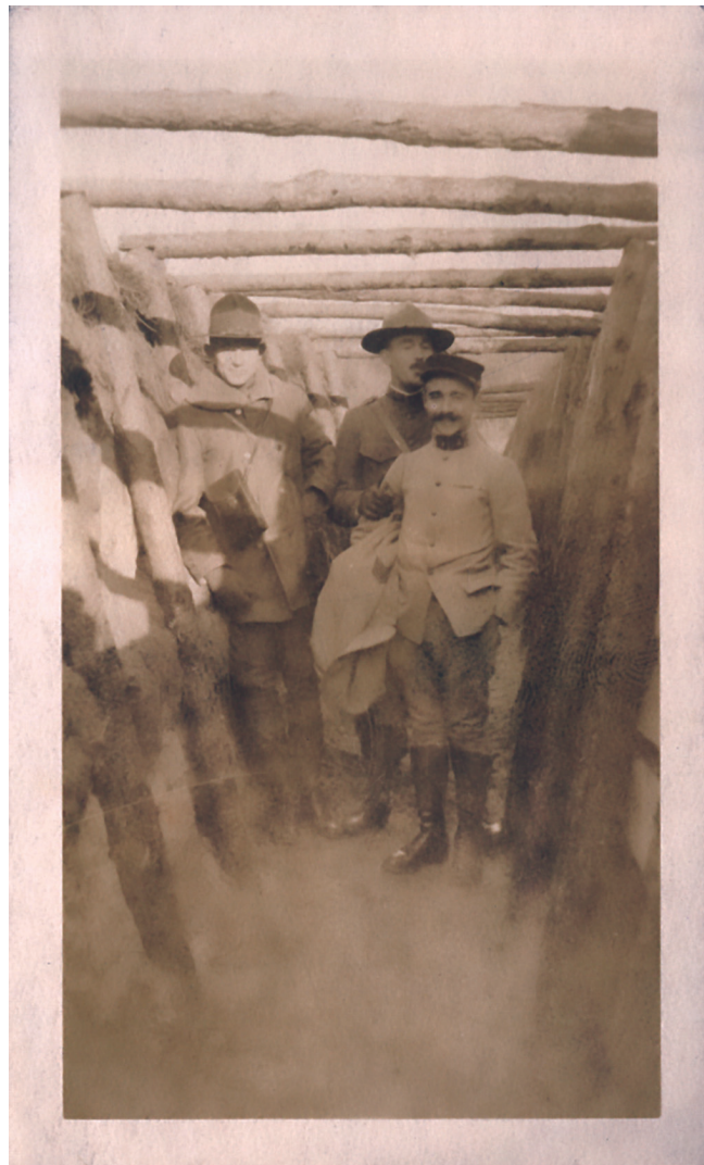
Speed (on left) in a communication trench. At the front Speed was the 3rd Battalion's telephone officer, leading a team of men to lay and repair cable lines. Speed Photo Collection, The Filson Historical Society.
