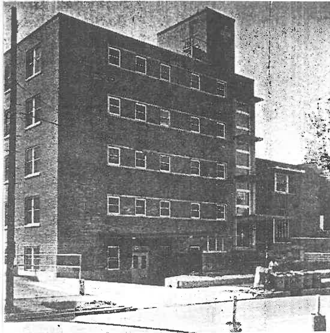
A NEW WING of Red Cross Hospital, 1436 S. Shelby, will be dedicated at an open house from 4 to 6 p.m. next Sunday. It is called the Alex Heyburn Memorial Building. Thomas J. Nolan & Sons, architects, designed it.
