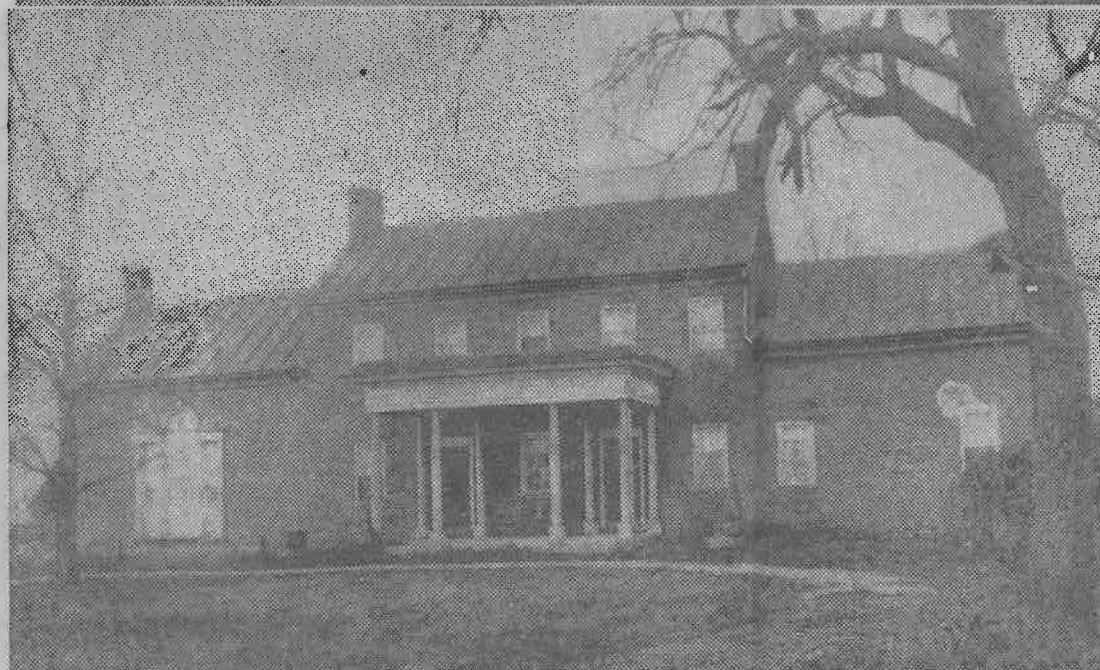
Pictures copied by Lafayette Studio Castlewood, at top, was built in Madison county in 1825 by James Estill, son of the hero of "Estill's Defeat." It is noted for its beautiful cabinet work and traditions of hospitality. Woodstock, below, representing an early and simple type of architecture, had a room added to the left just before the marriage of the daughter
