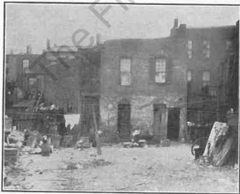
Wanted! A Tenement House Inspector
