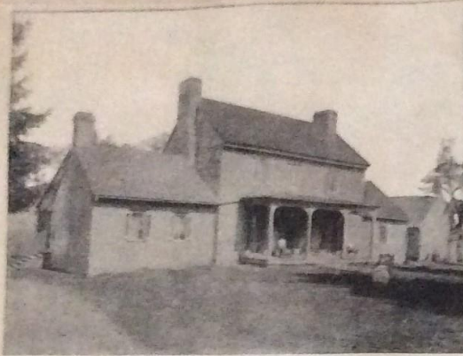
Traveller's Rest. (Front View.)
